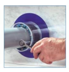
4. Tighten each bolt on each pressure plate about 2-3 turns, going around the pipe (do not cross-tighten bolts) until a proper seal is formed. A socket or offset wrench for 5/16, 1/2, 3/8, 9/16, 3/4, or 1-13/16" bolts will handle all installations.
