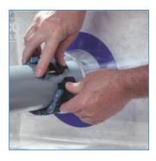
2. Wrap the PEN-SEAL around the pipe and connect the ends.
