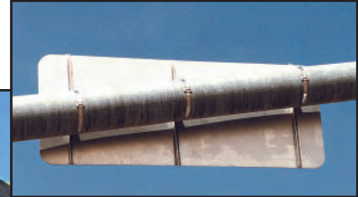
Mast Arm Sign Installation
