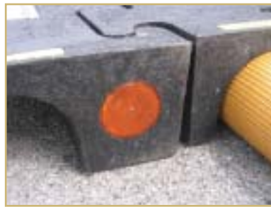
Recessed reflector on side of bridge warns approaching traffic
