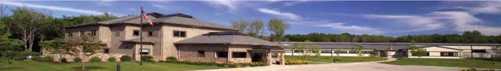
Snap-tite's Corporate Office and one of six manufacturing facilities centrally located near Erie, Pennsylvania, USA.
