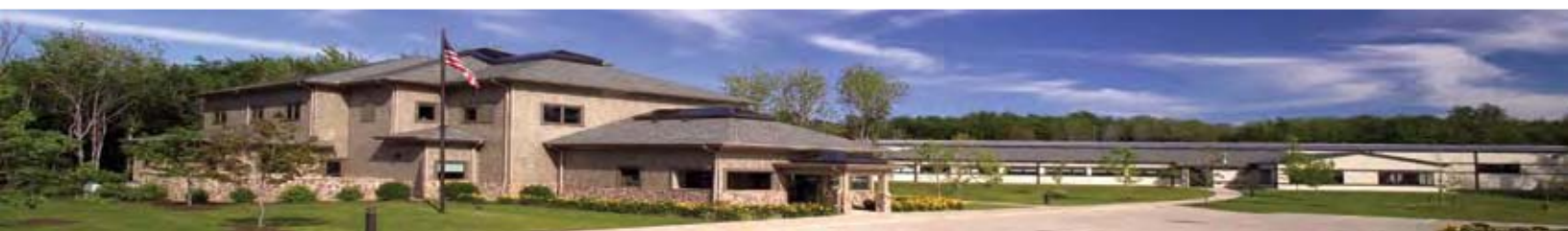
Snap-tite's Corporate Office and one of six manufacturing facilities centrally located near Erie, Pennsylvania, USA.
